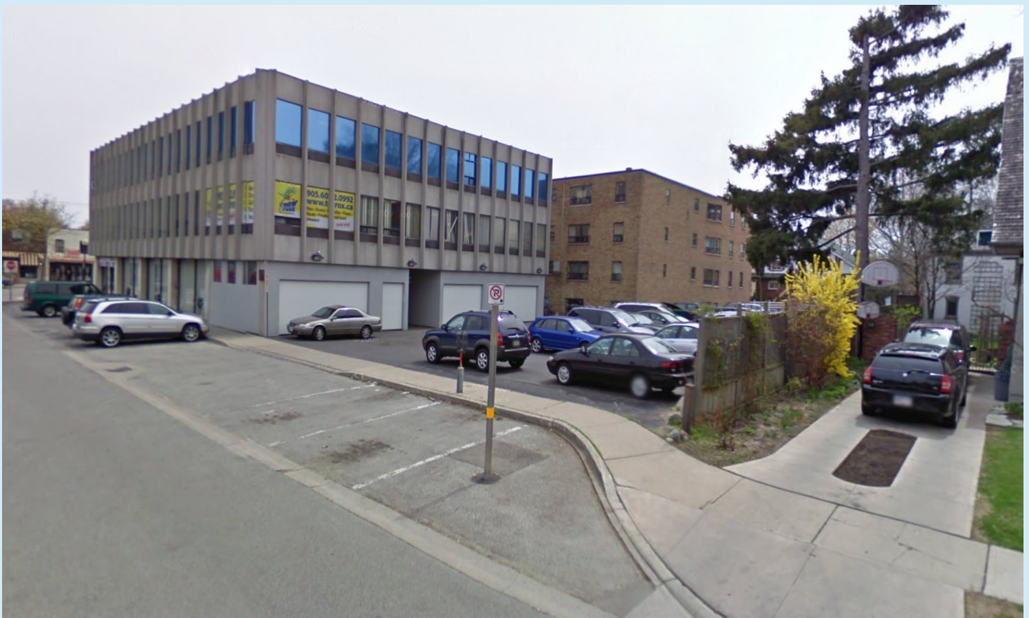
Figure C50 — Briarwood Avenue north of Lakeshore Road East
