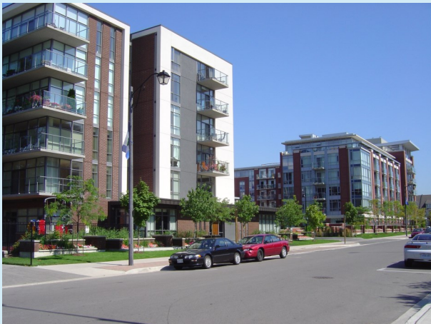
Figure B89 — Port Street East
