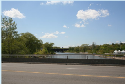
Figure B125 — Credit River
