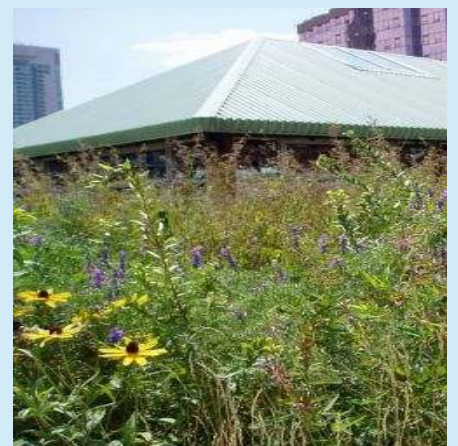
Figure D4 — Extensive' Green Roof, Mountain Coop, Toronto
