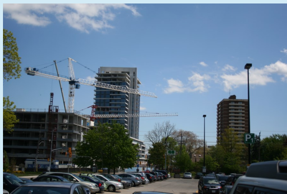
Figure B40 — Go Transit Lands parking lot looking south. Floor plate of the Northshore building is 964 m 2 (as defined under GFA)
